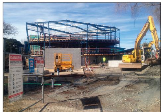
Boulder 2 later in the programme, with purlins being installed on the roof.
