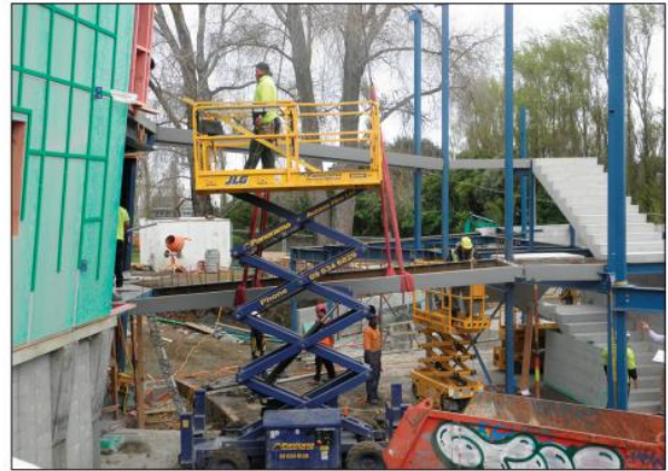
The walkways connecting Boulders 1 and 2, and the men who use scissor lifts to cut through the visual clutter.
