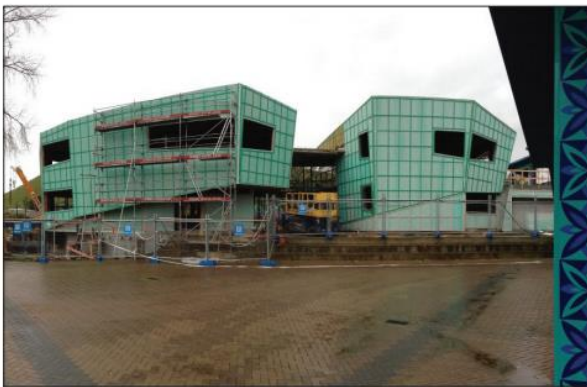
Boulders 2 and 3, covered in RAB Board, which forms the inside wall of the cavity system that allows for drainage. Longrun steel will be used for the exterior cladding.
