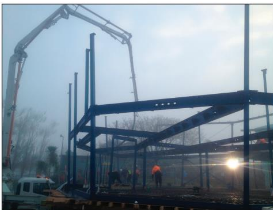
At Boulder 2, concrete is poured in early morning mist.
