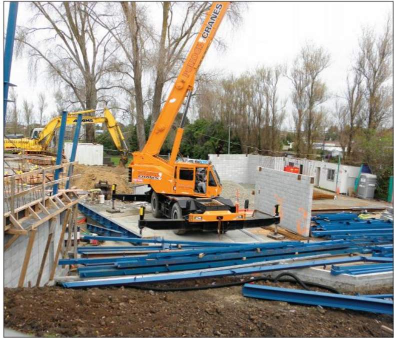
Continued page 24 A rough terrain crane operating in the constrained setting down space.
