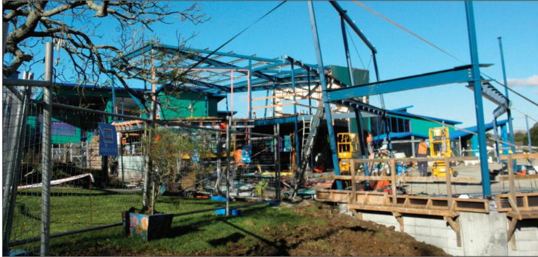
Temporary straps hold tilted columns in position pending bolt up.
